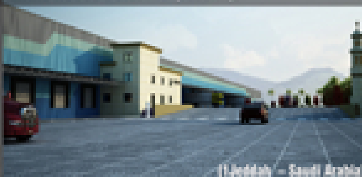
WARE HOUSE BUILDING (JEDDAH).
